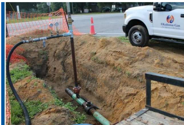
The vacuum purge system was attached to the new section of steel pipe - attached to the purge stack - and a vacuum was created in the new pipe down to approximately 14.5 psig
