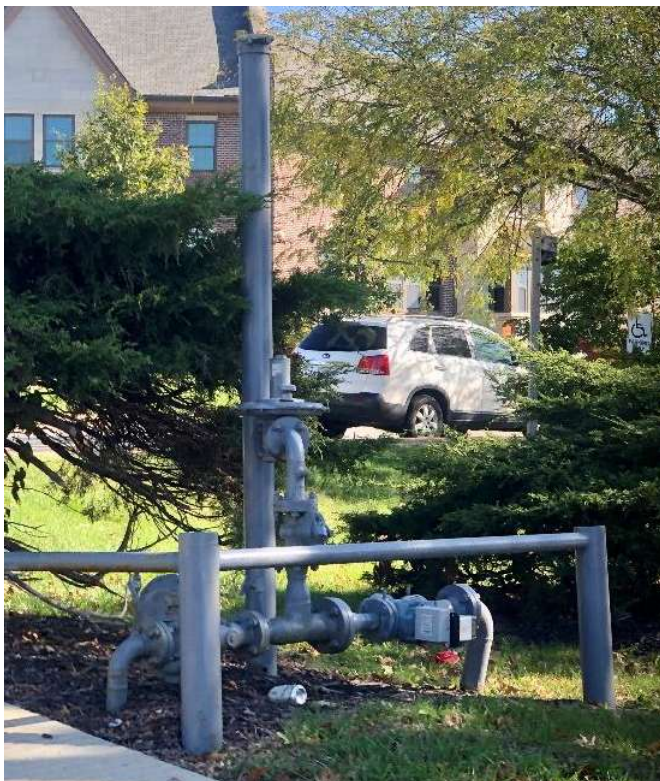
Relief Valve Assembly
