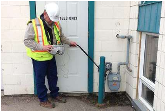
Field inspection of gas service equipment using leak detection technology
