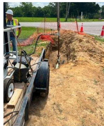
The vacuum purge system was attached to the new section of steel pipe - attached to the purge stack - and a vacuum was created in the new pipe down to approximately 14.5 psig
