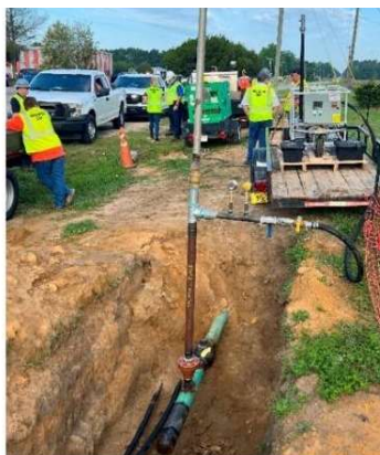
The vacuum purge system was attached to the new section of steel pipe - attached to the purge stack - and a vacuum was created in the new pipe down to approximately 14.5 psig
