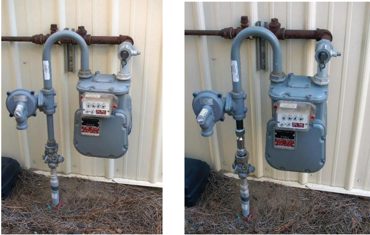
Figure 1. Meter set before and after the installation of the breakaway fitting
