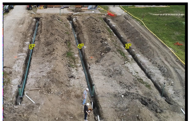
'Pipe farm' with open trench pipe installation
