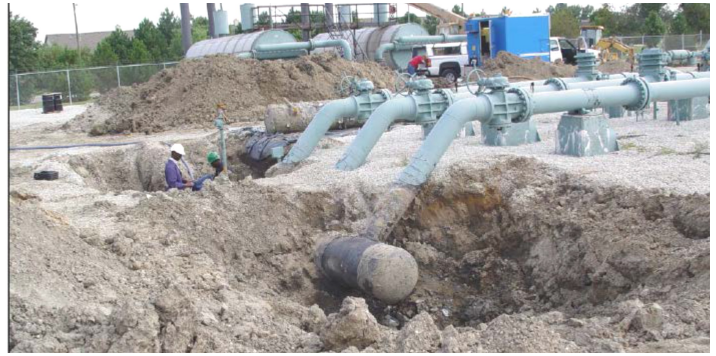
Congested meter-regulator station DA site with tees, stubs, and tap lines.
