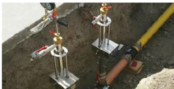
Figure 1. Kleiss stopper system controlling system flow on PE piping systems
