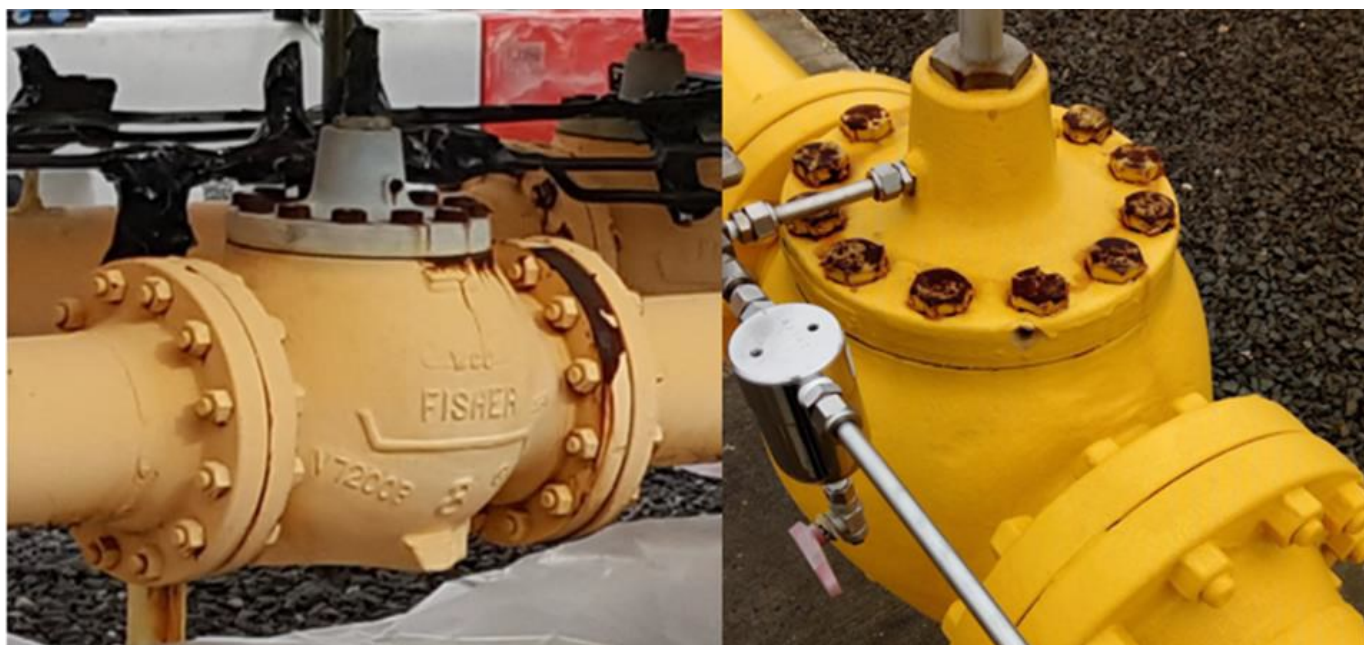
Regulator bolt rust in November 2015 (left) and in April 2017 (right).
