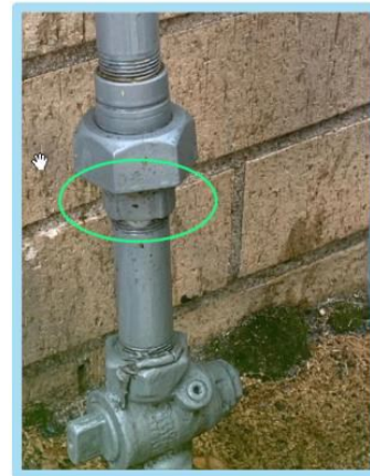
The meter has a small leak 200 ppmXm below the insulated union
