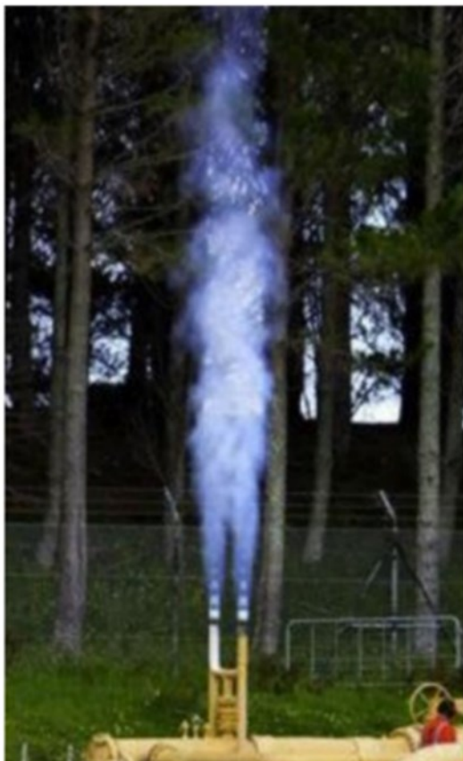
Figure 1: Pipeline purging operation
