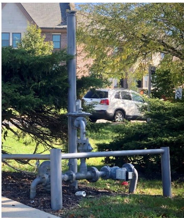
Relief Valve Assembly
