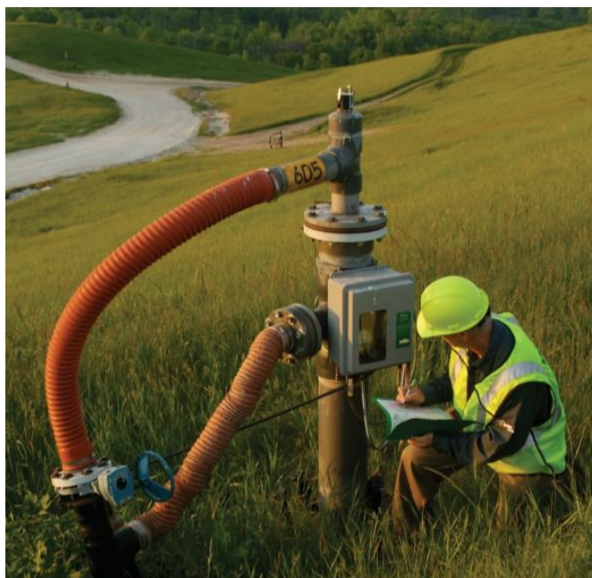
Landfill Gas Collection Wellhead
