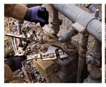
creating downstream gas leaks on customer piping due to the excessive stress and strain created from pipewrenching activities required to un-seize these fittings. This tool will improve employee and customer safety along with reducing time required to repair customer piping leaks created by during routine meter changes and removals.
