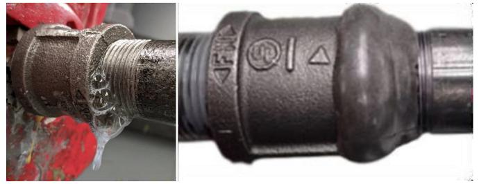
Left: Leak detection size of bubbles prior to repair; right: example of repaired leak after putty is applied.
