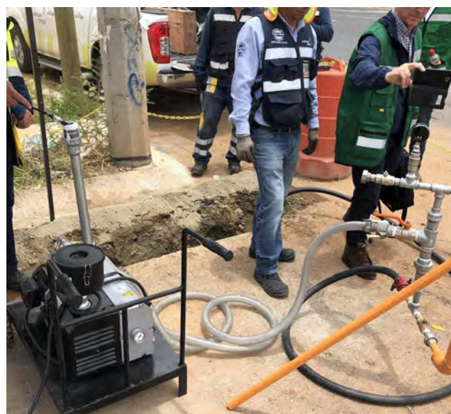
A utility crew purging a section of pipe using vacuum instead of venting gas to the atmosphere.
