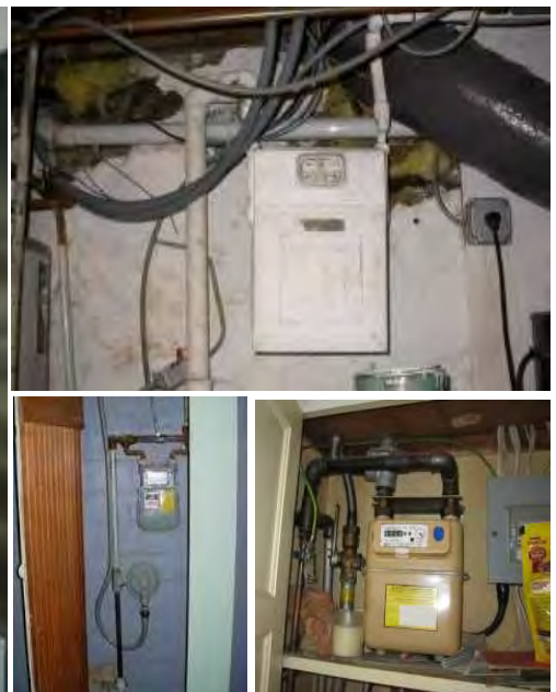
Gas meters installed indoors can present significant challenges for gas utilities.
