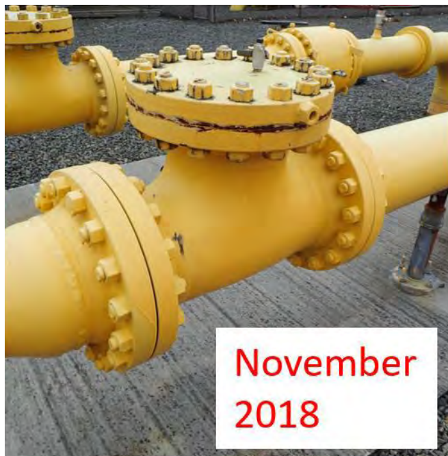
Comparison of polyurea coating between April 2017 (left) and November 2018 (right).
