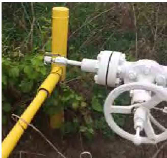
Gas sampling point at underground natural gas storage wellhead.
