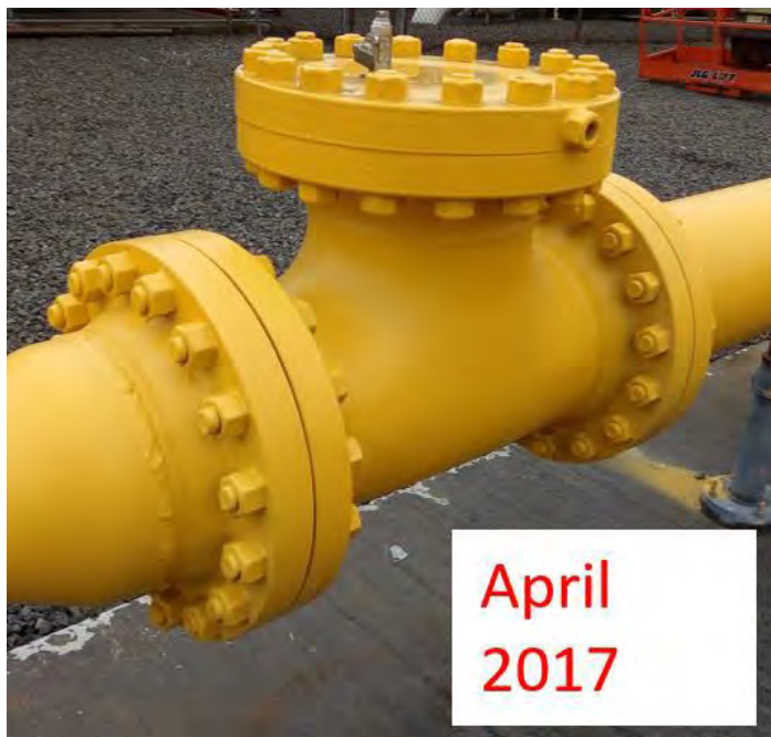
Comparison of polyurea coating between April 2017 (left) and November 2018 (right).
