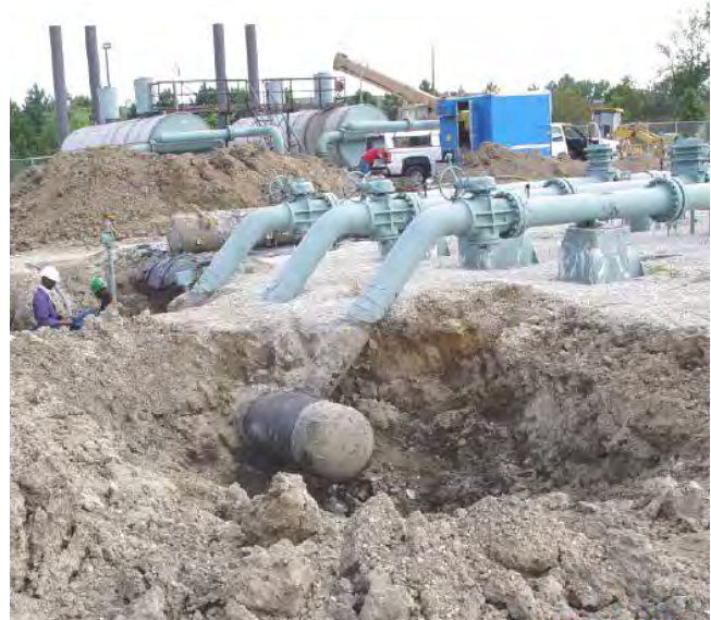
Congested meter-regulator station DA site with tees, stubs, and tap lines.
