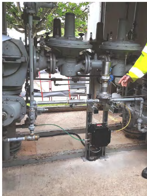
Pressure regulator station with Utonomy Smart Regulator installed.
