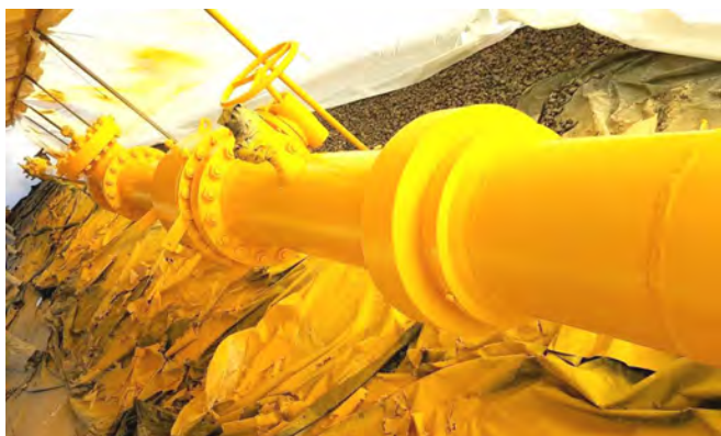
Pipe after application of polyurea coating and paint (November 2015).
