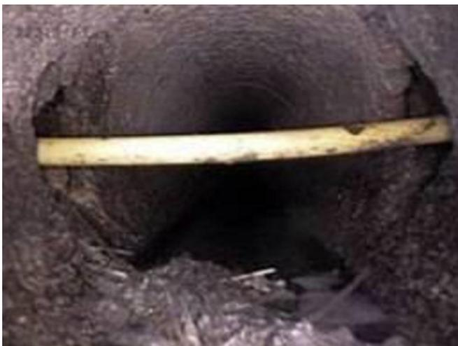
**A cross bore is defined as an intersection of an existing underground utility or underground structure by a second utility installed using trenchless technology resulting in direct contact between the transactions of the utilities compromising the integrity of either utility or underground structure.**
