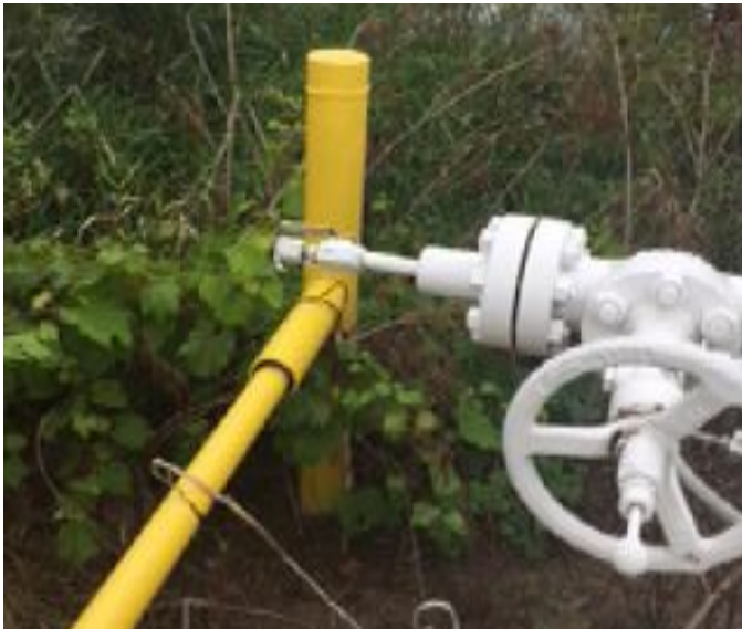
Gas sampling point at underground natural gas storage wellhead.
