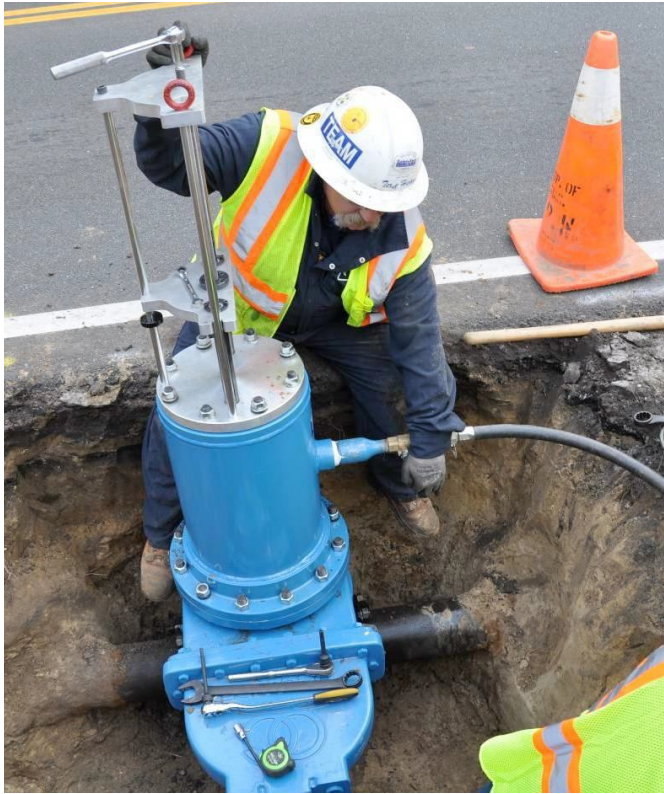
Field use of water industry cut-in valve.
