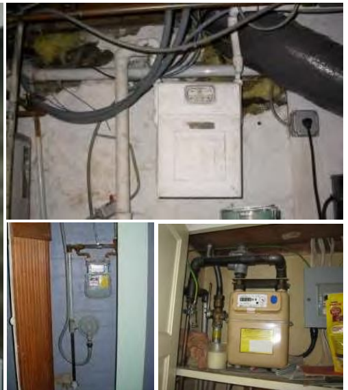
Gas meters installed indoors can present significant challenges for gas utilities.
