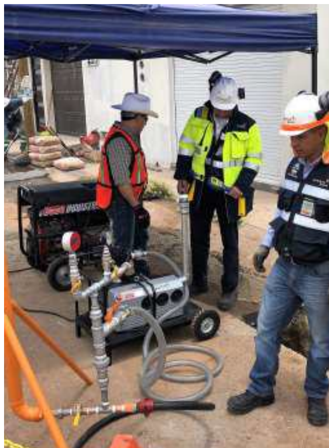
A utility crew purging in a section of pipe using vacuum instead of venting gas to the atmosphere.
