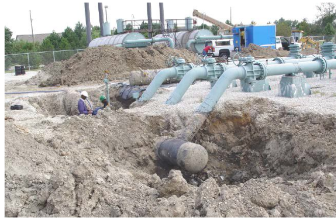
Congested meter-regulator station DA site with tees, stubs, and tap lines.
