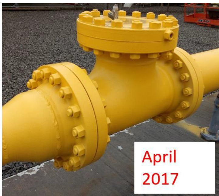
Comparison of polyurea coating between April 2017 (left) and November 2018 (right).
