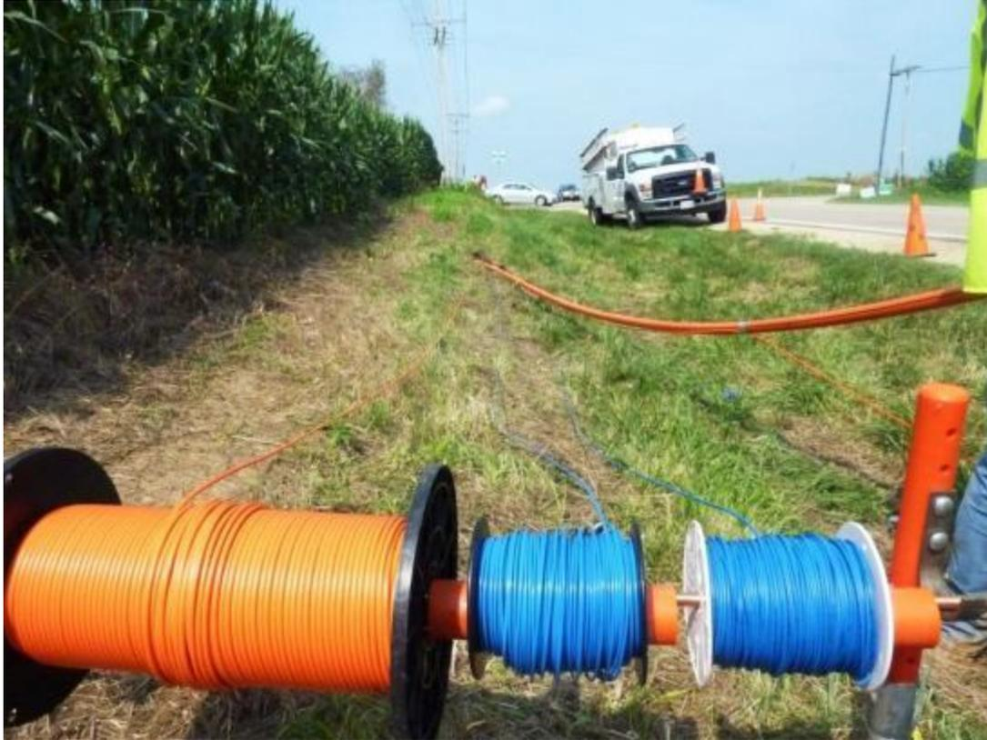
**Figure 45. Tracer Wires during Pull In**
