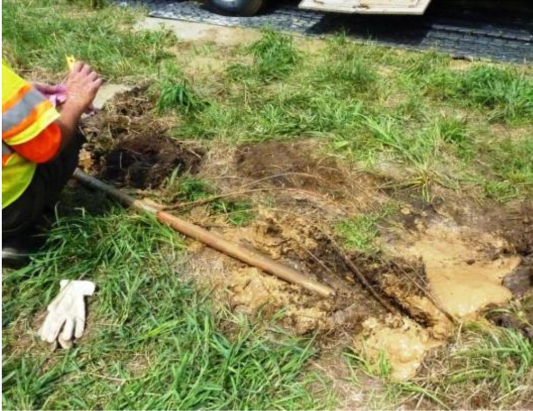
**Figure 47. Tracer Wires and Pipe at Exit Point (530' away from Entry Point)**
