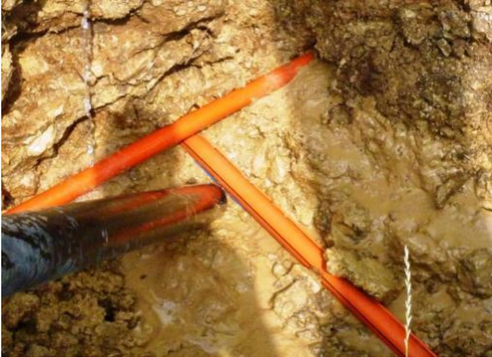
**Figure 46. Pipe and Wires Crossing Another Existing Conduit**
