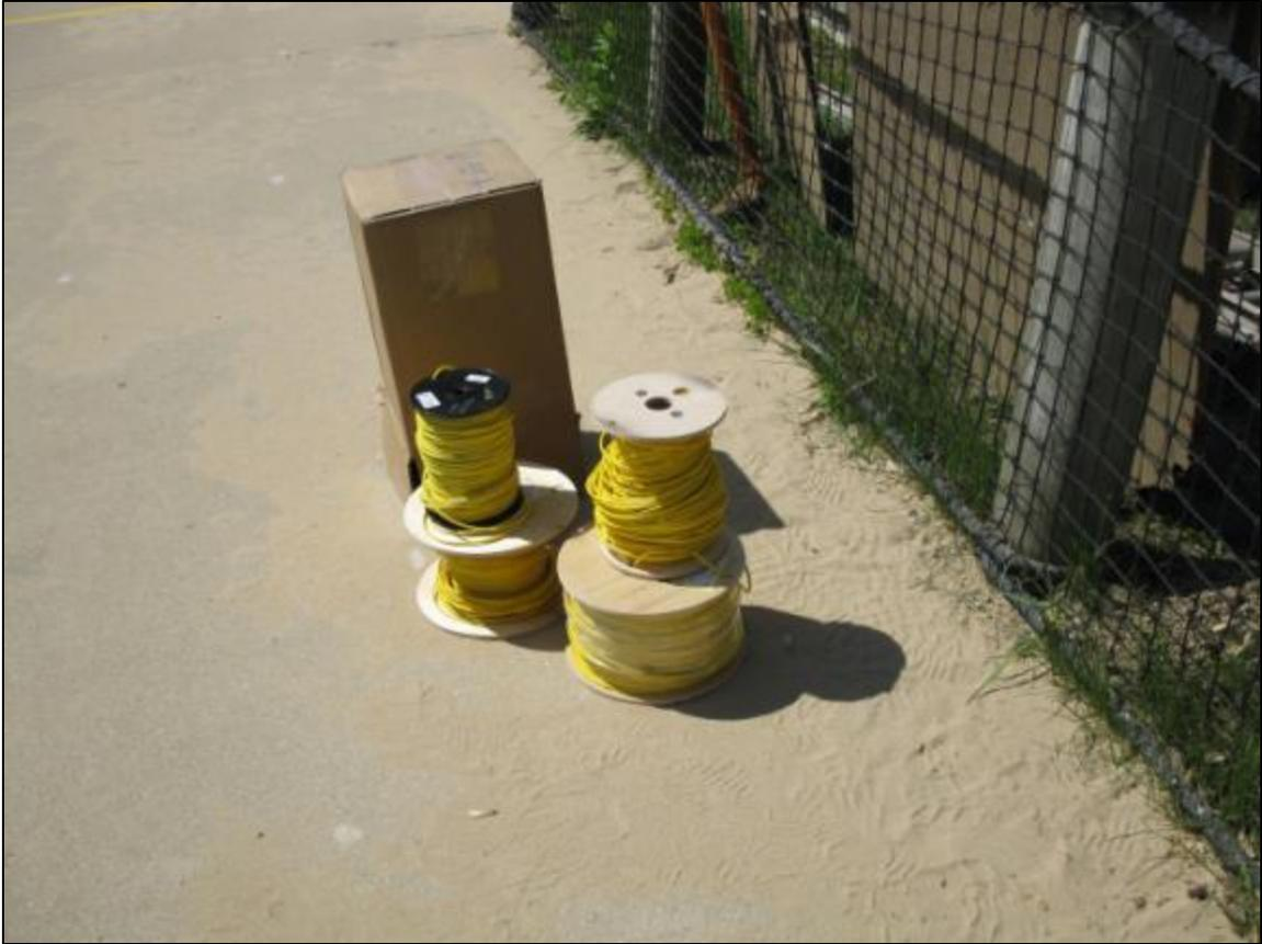
**Figure 51. Tracer Wires before the Installation**
