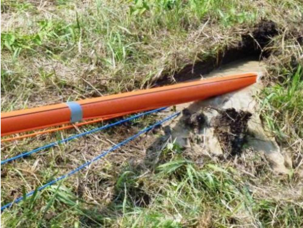
**Figure 44. Tracer Wires being Pulled in with Pipe**
