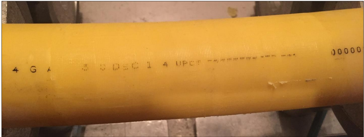
Figure 15. Typical scrape by 2" IPS Half-Moon Scraper (after several passes)
